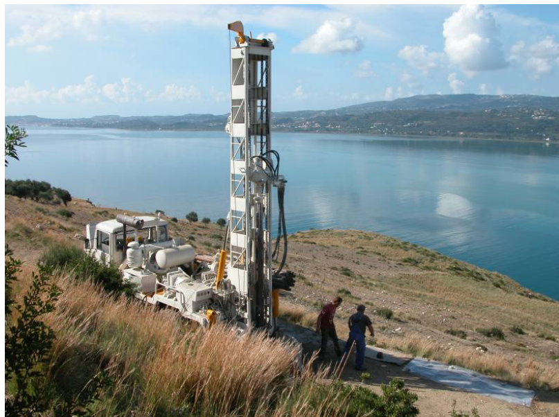
Figure 1: Drilling the 122 metre (400 foot) test borehole No solid limestone bedrock was encountered between the surface and sea level
